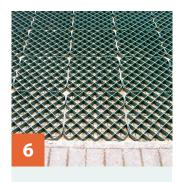
Ensure all the GroundGuard tiles are secure and the spikes are pressed into the ground.
