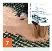
Finally, fill the tiles with any mixture suitable for seeding grass or gravel.
