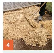
Put down an even layer of 2cm deep compacted sand on the area.
